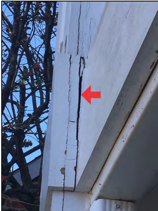
19. Caulking missing or deteriorated
