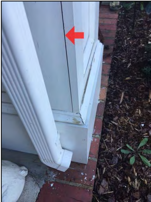
23. Caulking missing or deteriorated
