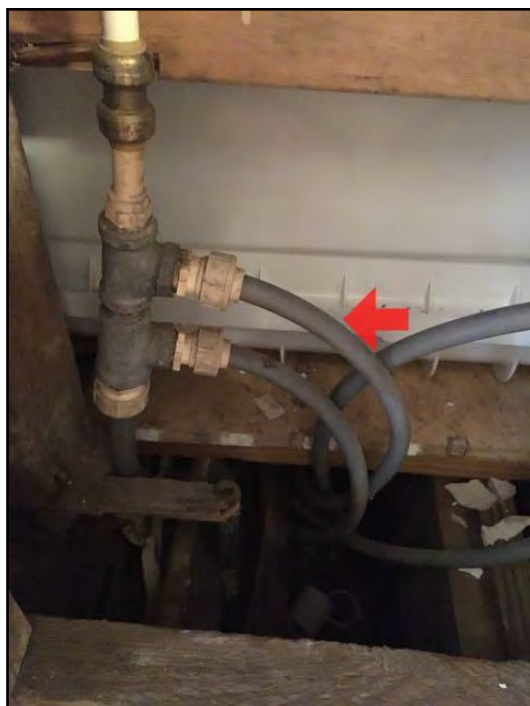
50. Suspect polybutylene connections
