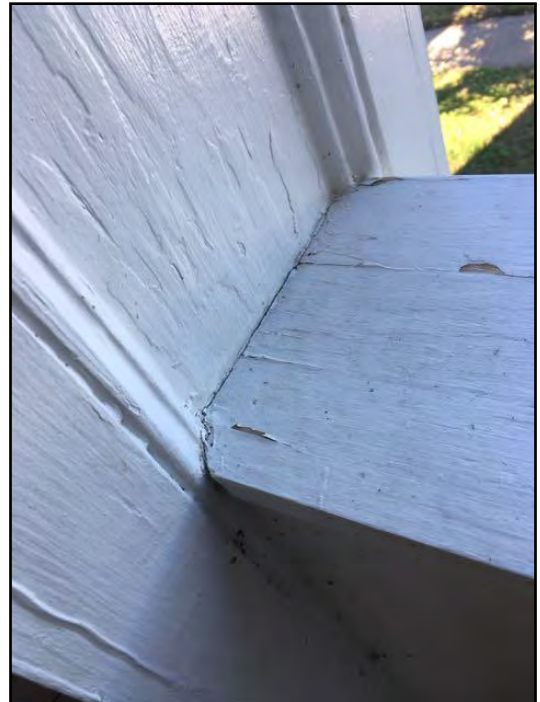
24. Caulking missing or deteriorated
