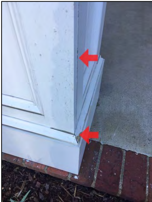
17. Caulking missing or deteriorated
