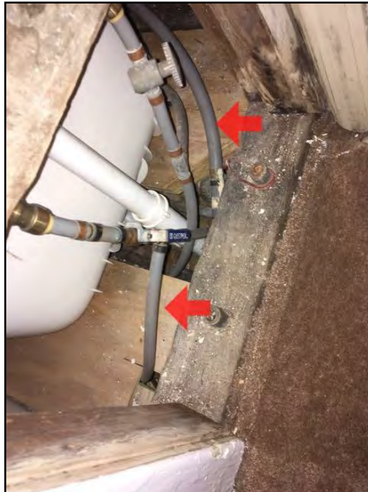
52. Suspect polybutylene connections
