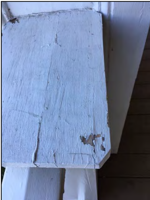
29. Caulking missing or deteriorated
