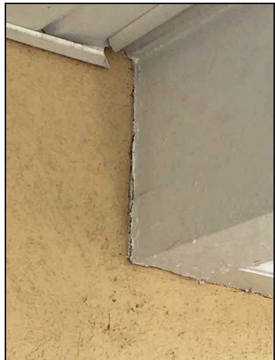
33. Caulking missing or deteriorated
