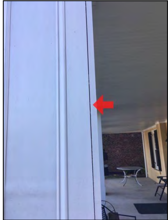
12. Caulking missing or deteriorated
