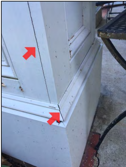
21. Caulking missing or deteriorated
