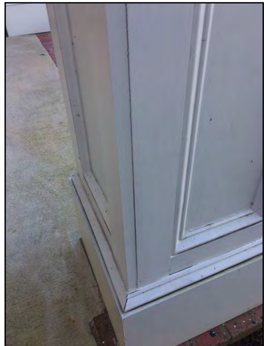
14. Caulking missing or deteriorated
