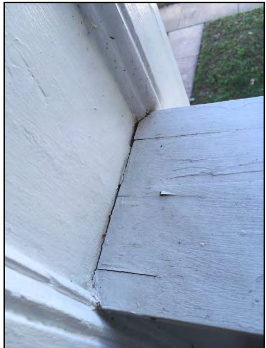
30. Caulking missing or deteriorated
