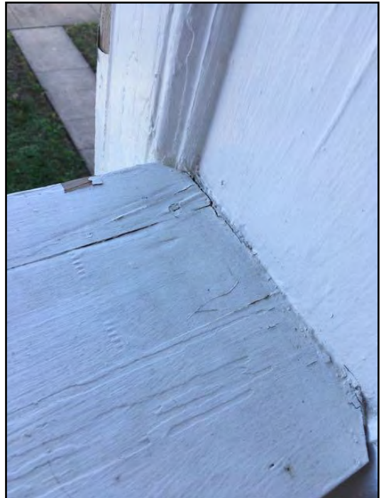
28. Caulking missing or deteriorated
