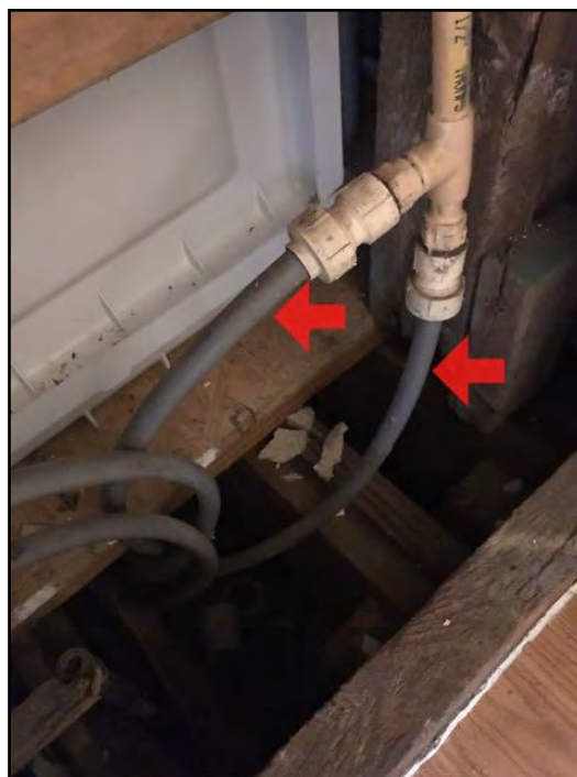
51. Suspect polybutylene connections
