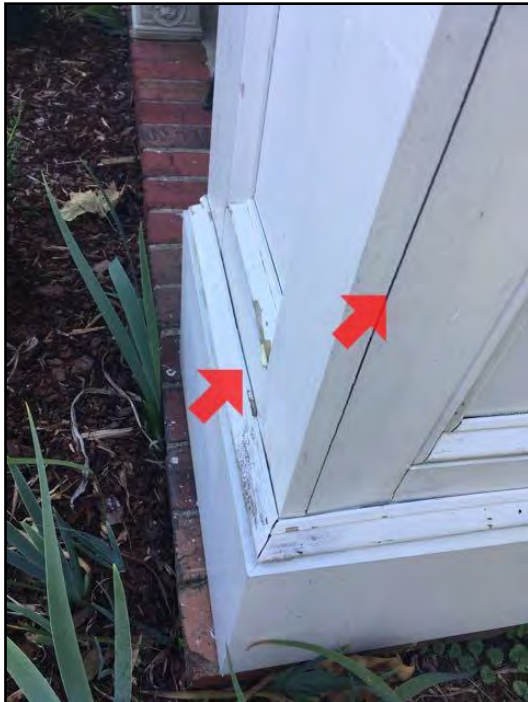
15. Caulking missing or deteriorated
