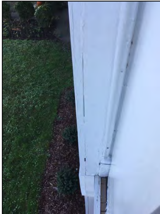
31. Caulking missing or deteriorated
