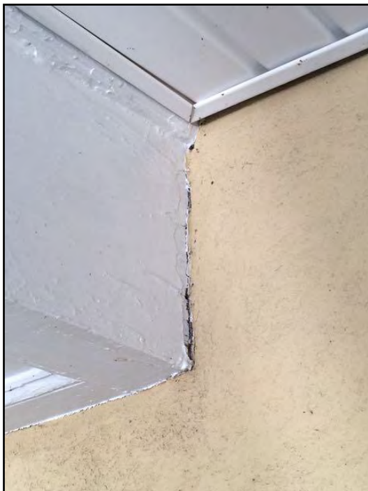
32. Caulking missing or deteriorated
