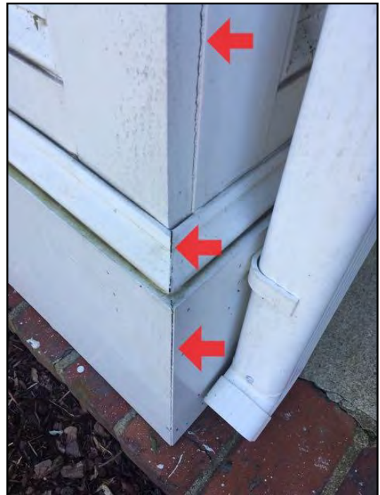
22. Caulking missing or deteriorated
