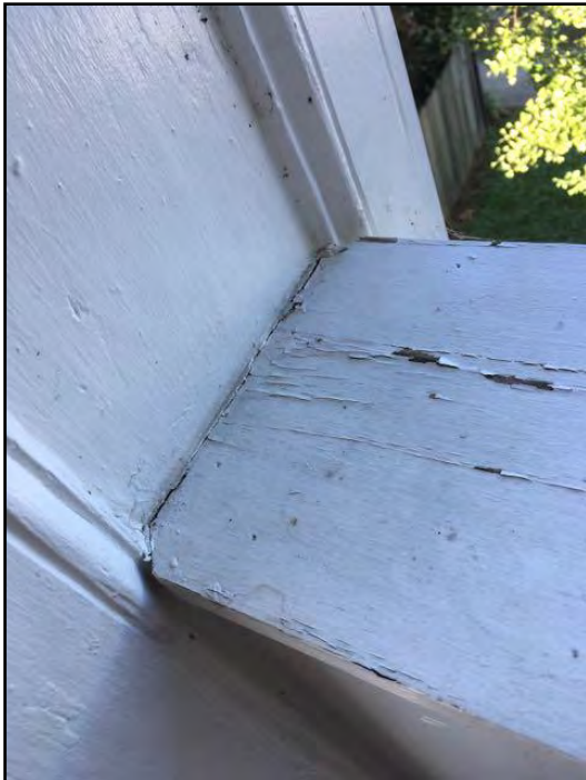
27. Caulking missing or deteriorated
