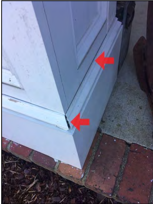
11. Caulking missing or deteriorated
