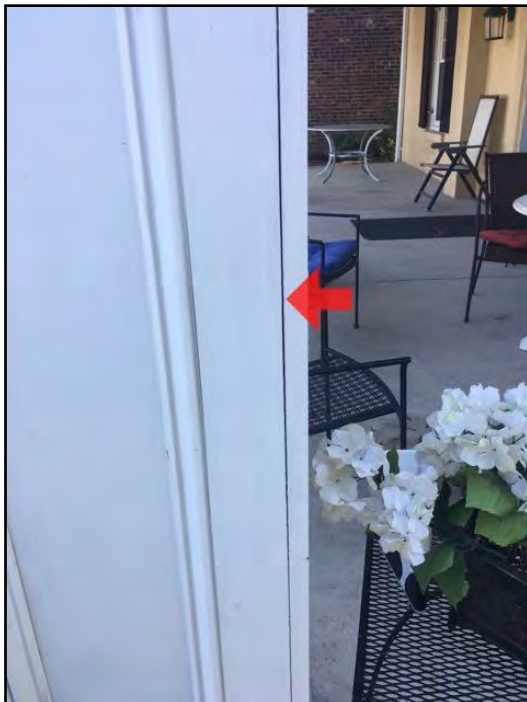
13. Caulking missing or deteriorated
