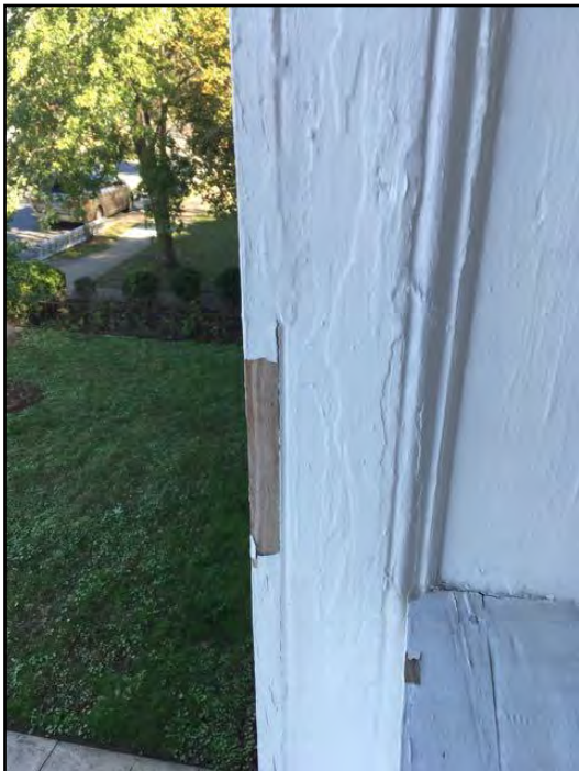
25. Caulking missing or deteriorated
