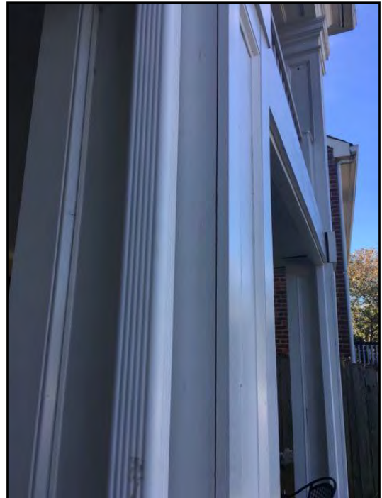
20. Caulking missing or deteriorated
